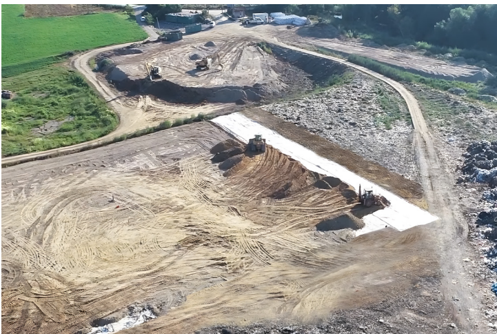
Large Pozidrain rolls enabled rapid installation
