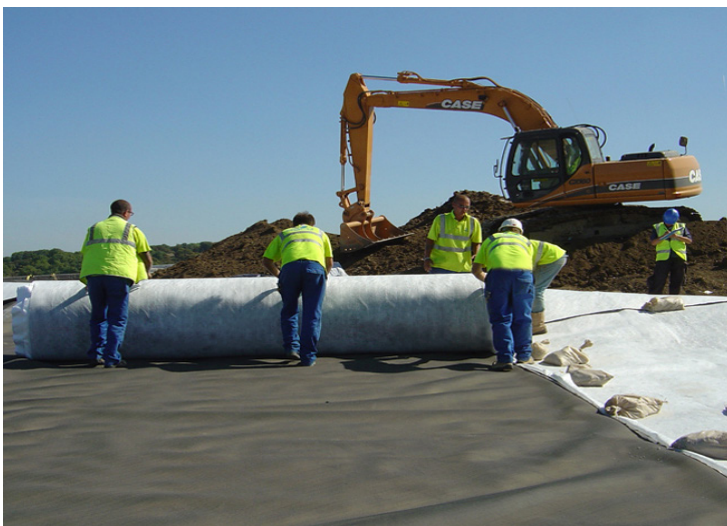
Pozidrain installed on top of 1mm LLDPE textured liner
