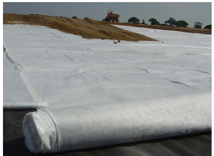
Adequate interface friction ensured slope stability
