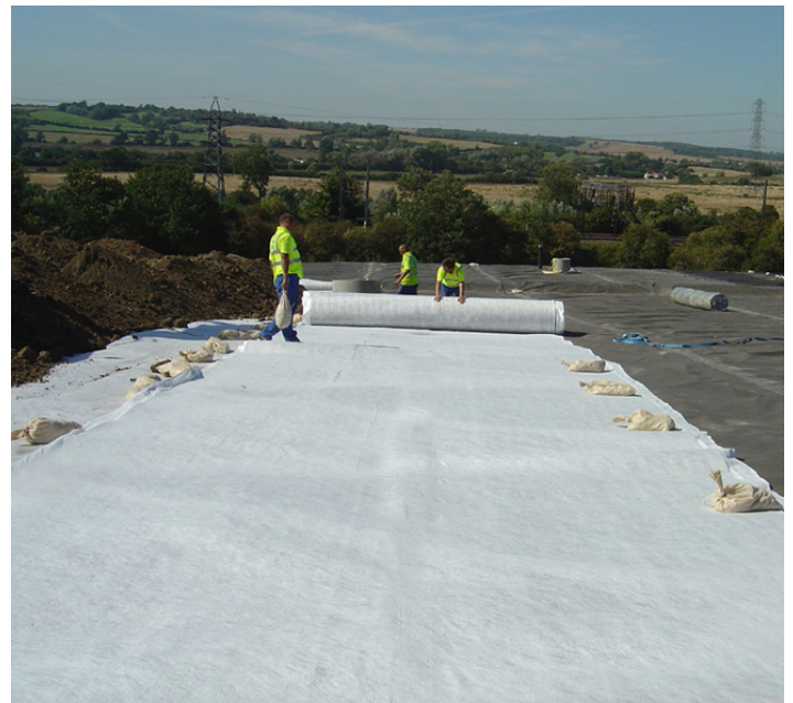
Large rolls enabled rapid installation
