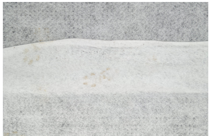
Overlap prevents soil ingress and holds panel in place
