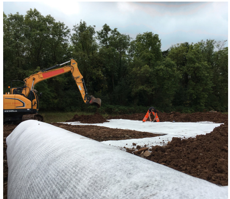
Backfill operation followed immediately behind the geotextile filter jointing
