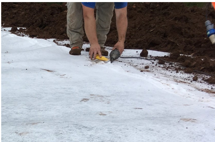
Simple heat weld joints on geotextile
