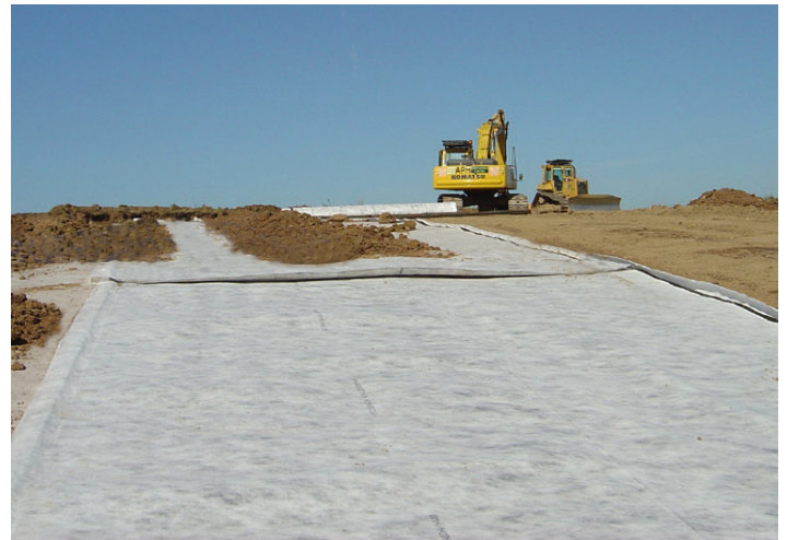
Large rolls enabled rapid installation
