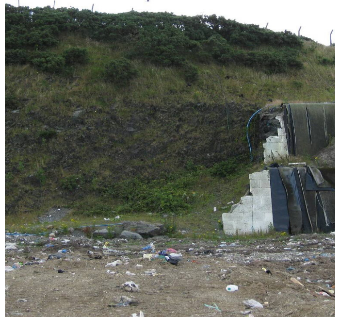
Steep Wall with lining system
