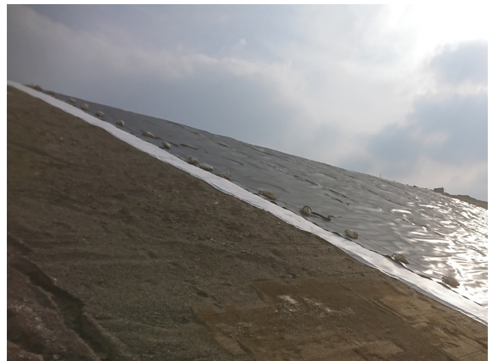
Long, wide rolls enabled fast installation
