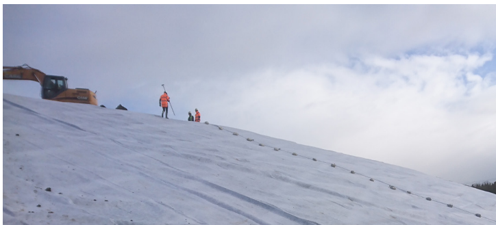
Pozidrain is stable on steep slopes of up to 1:2.5 (21.8%)
