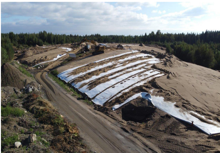
Deckdrain geocomposite on waterproofing membrane
