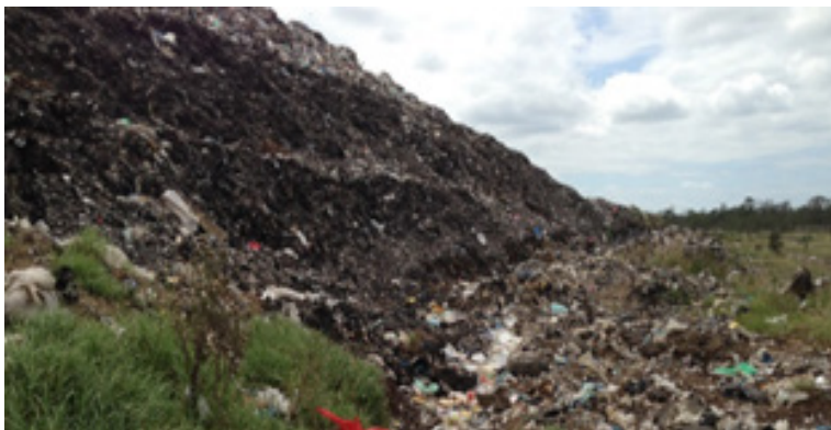
Old cells with unsafe, uncompact steep side slopes
