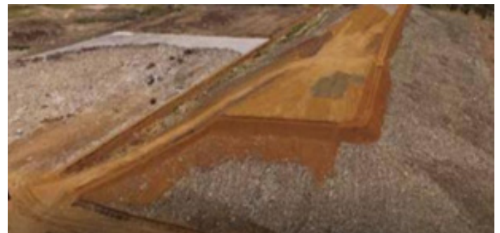
Reshaped cells 1 & 2 and start of temporary covering layer
