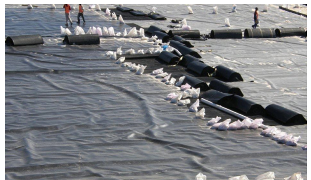
Fig. 7: Unused rolls used as ballast on flat areas
