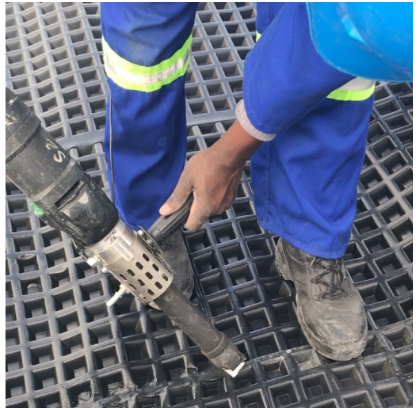
Fig. 10: Extrusion welding of joints (where Leakdrain supplied with a selvedge)
