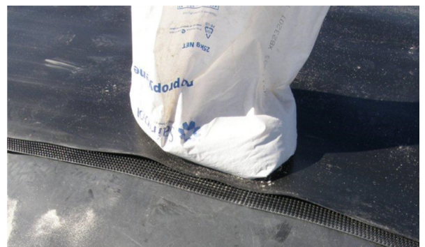
Fig. 6: Leakdrain installed dimple side up (example)
