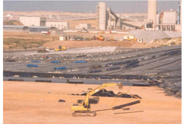
Fig. 5: Spreader beam carrying Leakdrain roll
