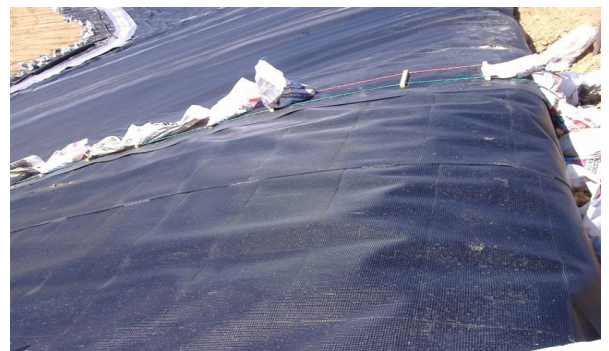
Fig. 8: Leakdrain folded into anchor trench
