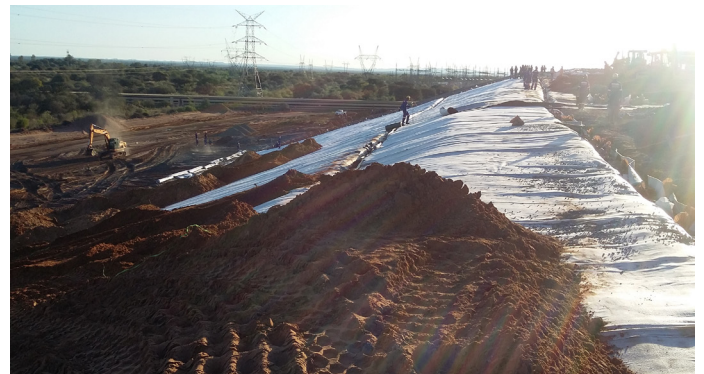
Pozidrain closing and draining the steep side slopes
