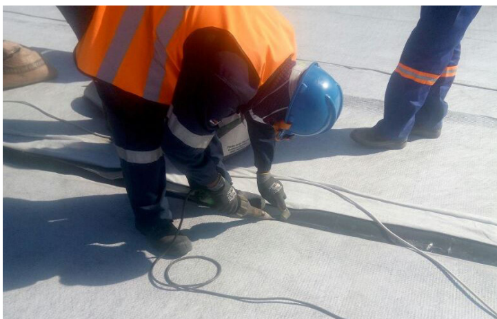
Hot air welding of the 100mm flat edges
