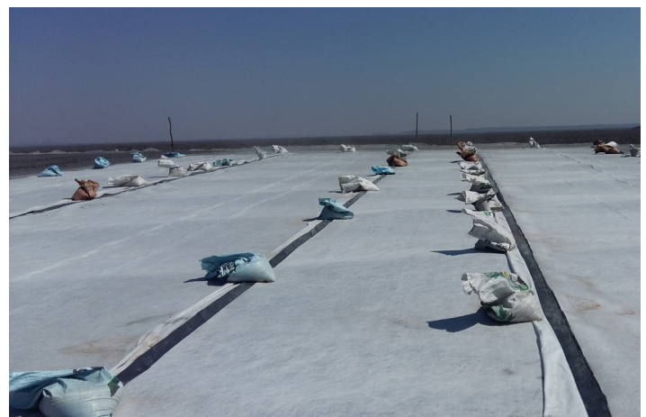
Welded seams awaiting inspection
