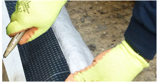
Fig. 4: Roll out and cut Piledrain to required length with safety knife.
