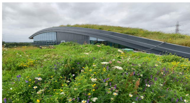
ABG Green Roof installation as part of a SuDS scheme
