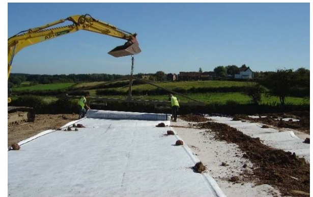
Fig. 6: Pozidrain All-in-One installation
