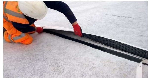
Fig. 9: Pozidrain K [L] Butt Joint with Butyl Tape
