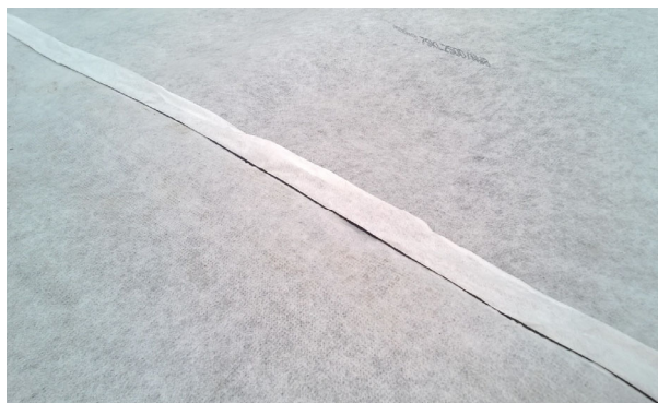
Fig. 10: Geotextile flap overlap
