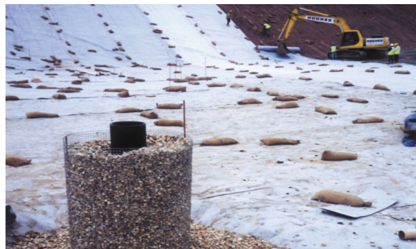
Fig. 7: Pozidrain basal drainage application
