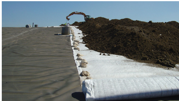
Fig. 6: Pozidrain placed on steep slope
