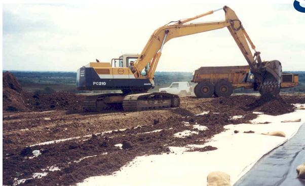
Fig. 14: Placing cover soil
