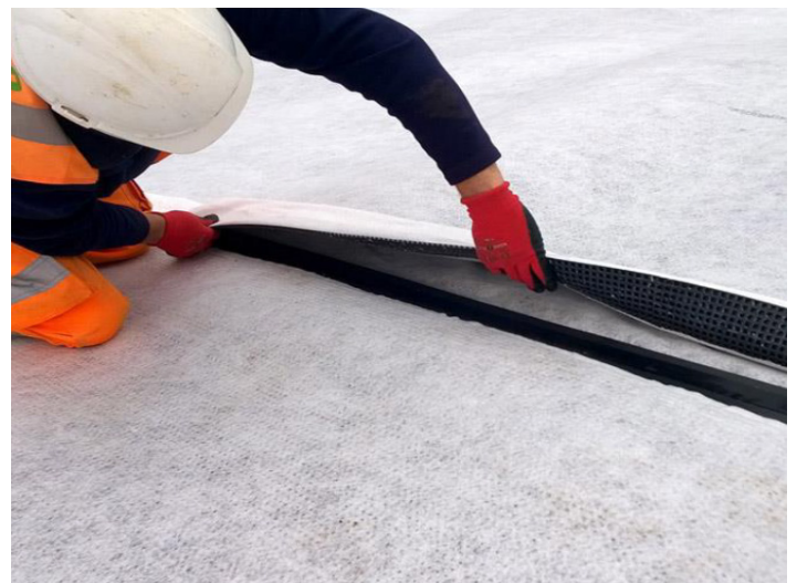
Pozidrain geocomposite flat selvedge overlapping and sealing with double sided Absel butyl tape
