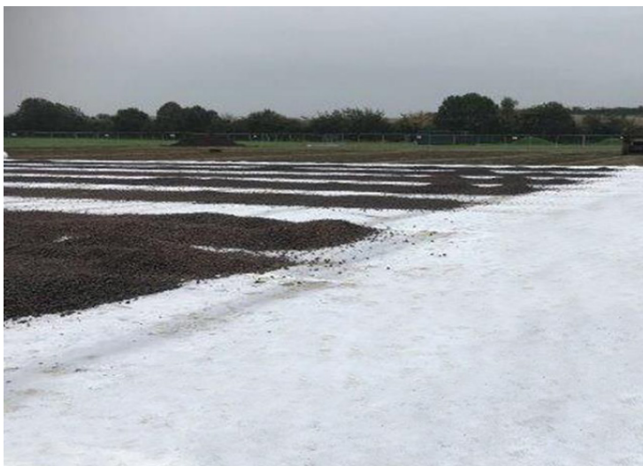
Large Pozidrain geocomposite rolls enabled rapid installation and replaced perforated pipes
