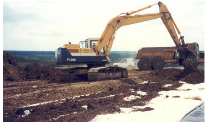
Fig. 14: Placing cover soil
