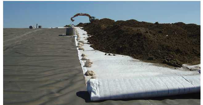
Fig. 6: Pozidrain placed on steep slope
