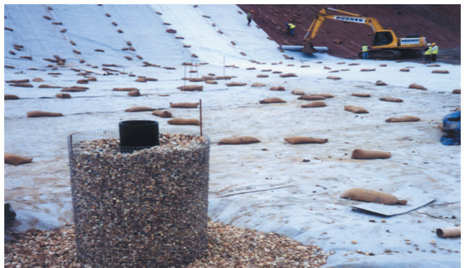
Fig. 7: Pozidrain basal drainage application
