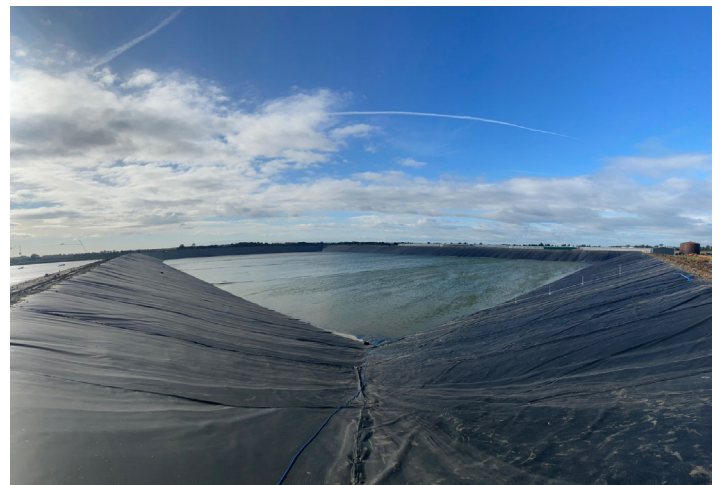
HDPE liner filling with water in the large 22 acre reservoir basin.
