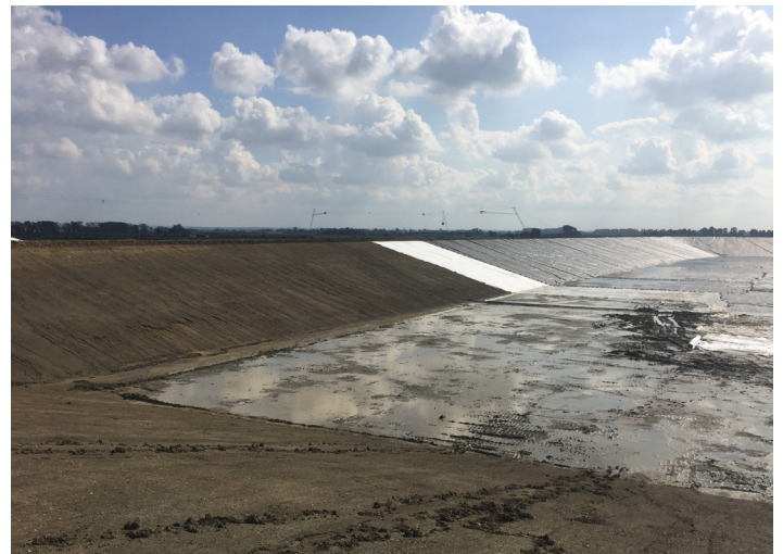
Terrex NW8 provides separation and filtration function to protect the integrity of the underlying soils
