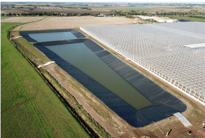
The 5.5 acre basin collects run-off from the adjacent greenhouse buildings and redirects it for irrigation of the crops.
