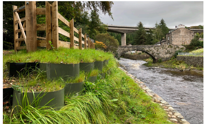
Webwall will eventually present a green finish
