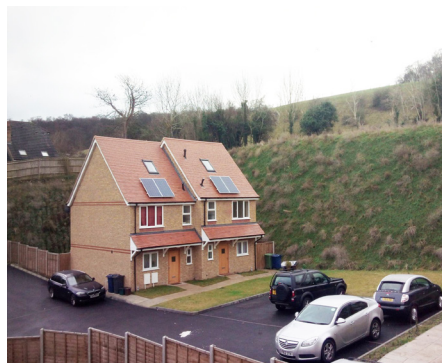
Webwall following initial grass coverage to provide a green finish
