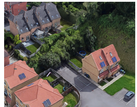
Webwall fully established following further growth / planting
