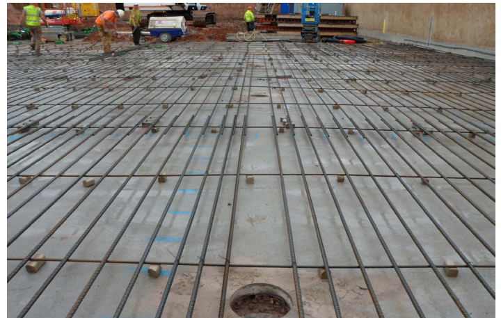
Reinforced floor slab preparation showing a valve position
