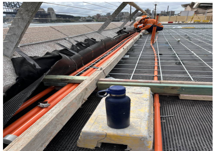
Cavidrain in position beneath concrete formwork
