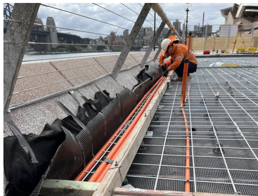
Cavidrain in position beneath concrete formwork
