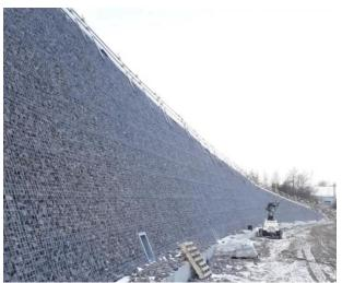
The finished SSTC rock/gabion style faced walls protected and drained with ABG Deckdrain.
