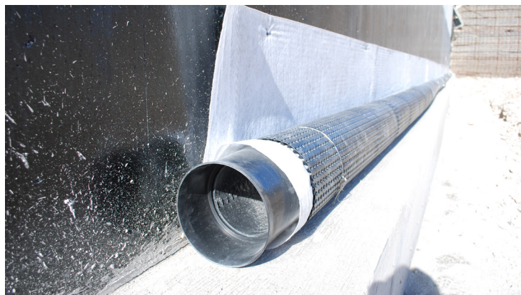
Deckdrain wrapped around a perforated carrier pipe
