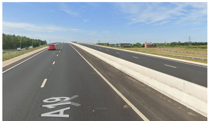
The completed A19 dual carriageway fly over structure
