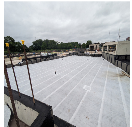
ABG Deckdrain being installed onto the podium deck roof areas
