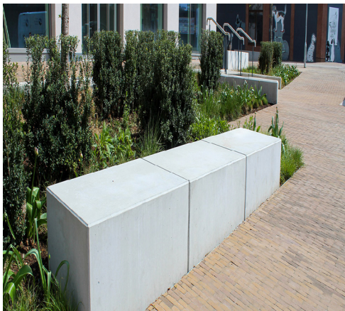
Completed area of podium deck landscaping with paving and planter finishes
