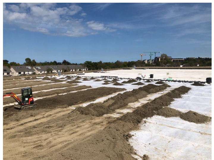
Placing of soil & growing media over the Pozidrain drainage layer
