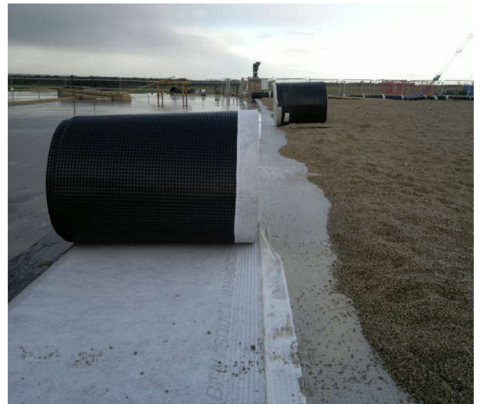
Deckdrain geocomposite with integral geotextile overlaps to create continuous drainage layer
