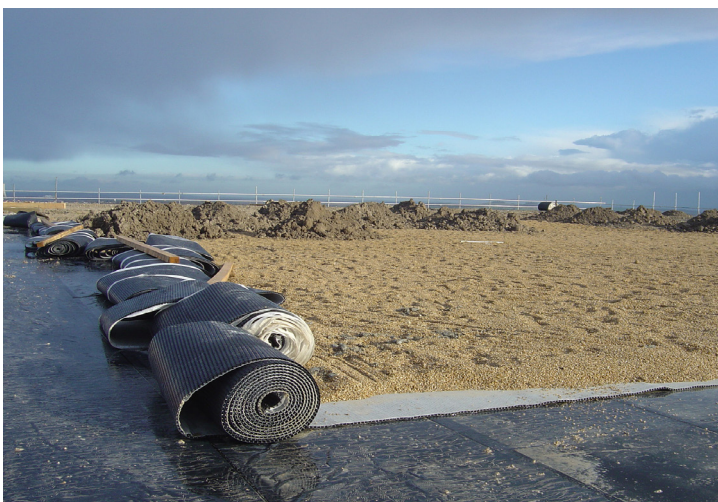
Deckdrain geocomposite on waterproofing membrane
