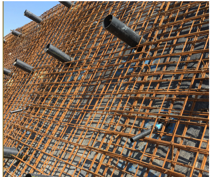
Deckdrain geocomposite, reinforcement and soil anchors Installation
