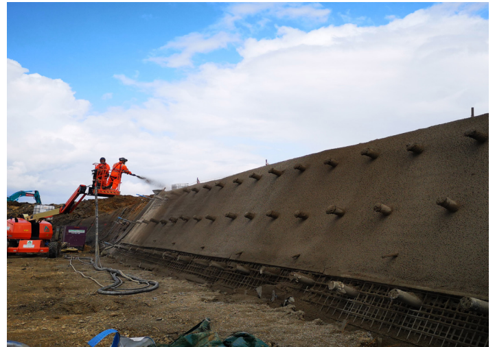
Shotcrete spraying on Deckdrain geocomposite
