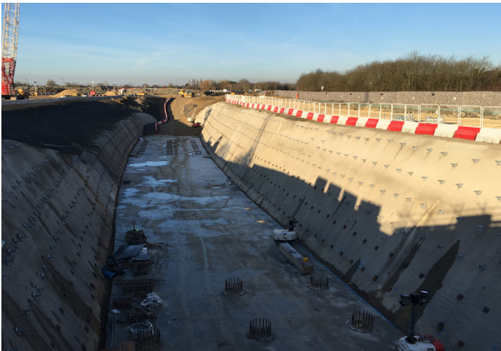
Completed retaining structure
