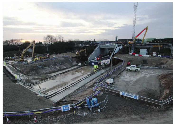
Bridge in final position with Deckdrain ready for fill
