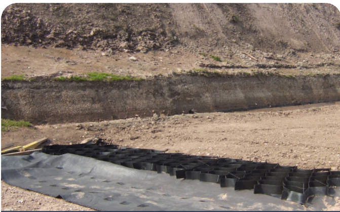
Geocell sub-base reinforcement over filter geotextile
