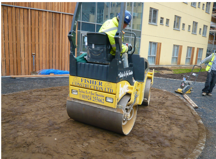
Controlled compaction of reinforced layer pre-turfing
