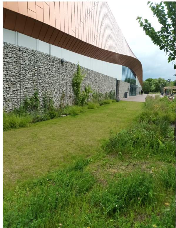
Natural reinforced grass access route around the perimeter of the Lee Valley Ice Centre
