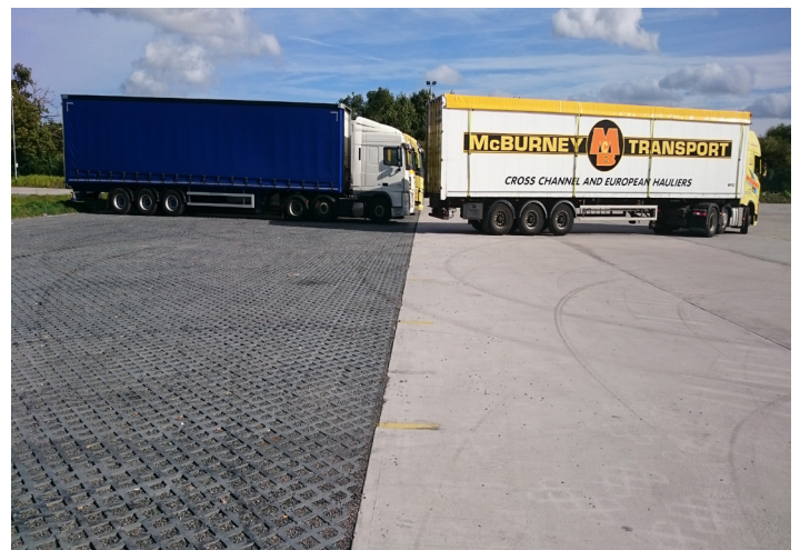
Designed for HGV braking, slewing and turning zones. Note the turning tyre marks caused by the HGVs
