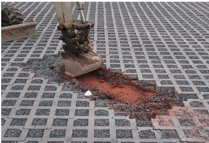
Easy to remove and relay for access to utilities
