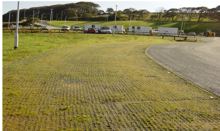
ABG Sudspave 40 is clipped together to create a continuous permeable reinforced surface. It is cut to fit the curving shape of the car park which fits the existing contours of the valley site.
