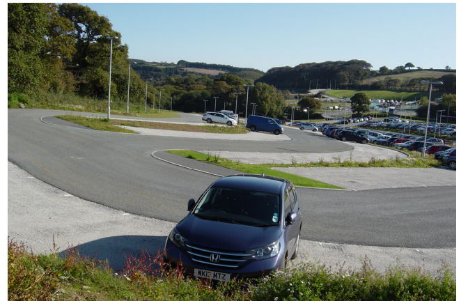
Gravel filled parking bays
