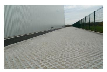
ABG's Truckcell 80 heavy-duty recycled permeable paving system installed to provide a durable, free-draining and long-term sustainable surface for this access route.
