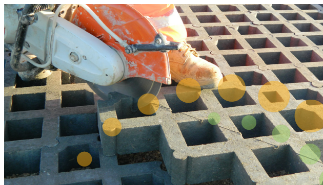
Cutting Truckcell to size
