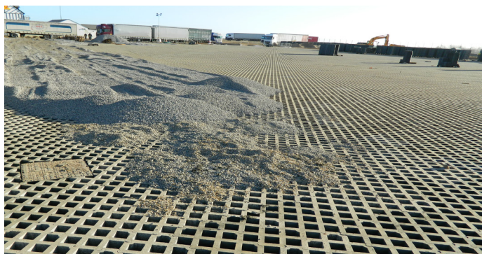
Truckcell being filled with porous angular aggregate
