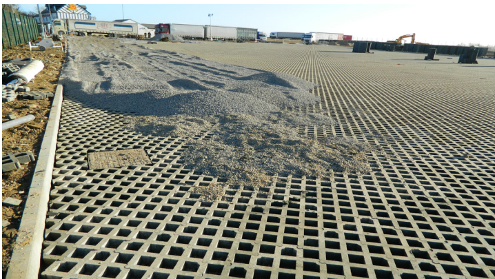
Truckcell being filled with porous angular aggregate
