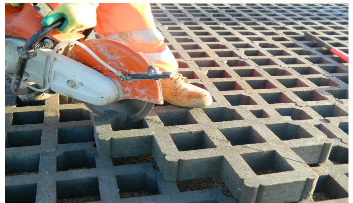
Cutting Truckcell to size
