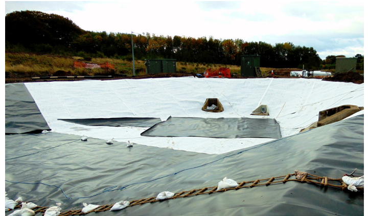
Pozidrain under the liner provides drainage, gas venting and puncture protection
