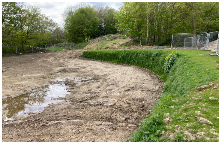
100m2 of Webwall installed for the Priory View SuDS pond scheme
