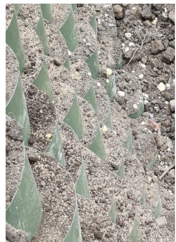
Type A panels to reach the retaining wall design height. Cells stepped back 100mm and filled with site won soils
