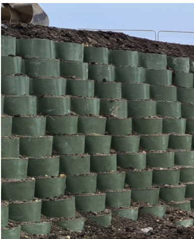
Type A panels to reach the retaining wall design height. Cells stepped back 100mm and filled with site won soils
