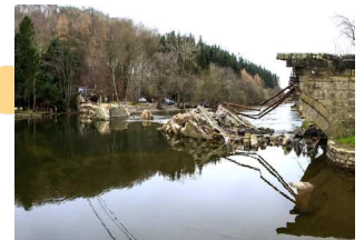
The former three arch stone bridge (left), washed away during Storm Desmond in December 2015 (right). The silty ground conditions prevalent on site required reinforcement prior to crane loadings.
