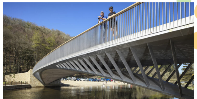
The new bridge in place with the working platform area suitable for car parking, visible in the background
