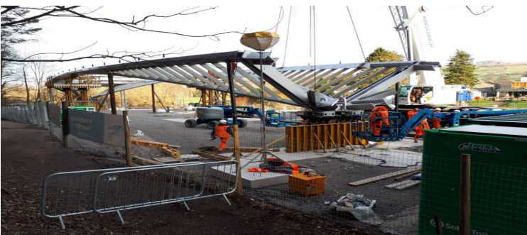
The steel span positioned ready for lifting on the working platform
