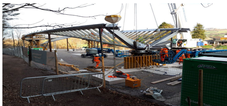
The steel span positioned ready for lifting on the working platform
