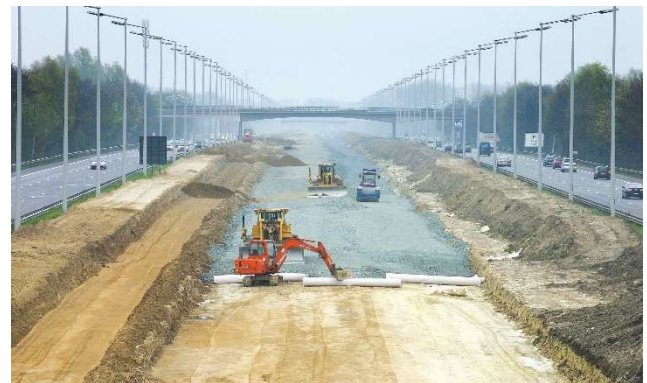
Fig. 2: Terrex nonwovens in road construction
