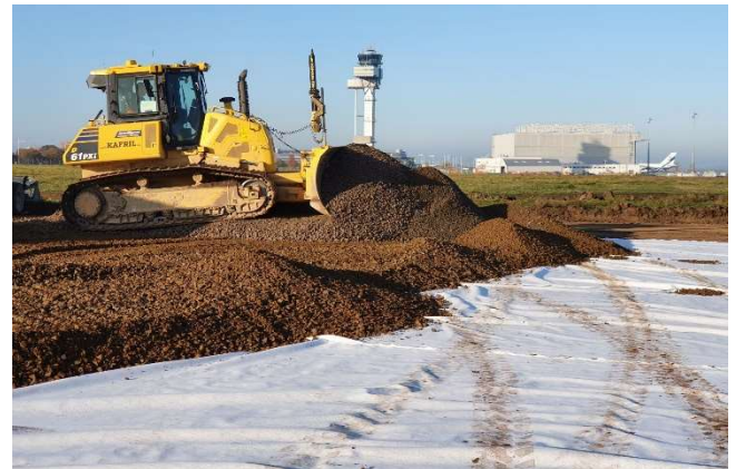
Fig. 7: Placement of backfill
