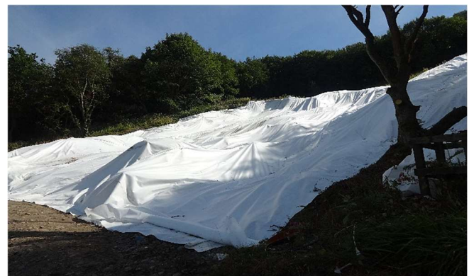
Fig. 8: Installation onto slopes for erosion control, conforming to dips / hollows
