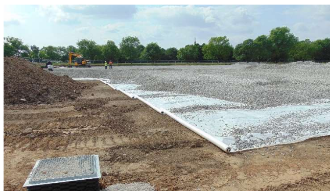
Fig. 5: Unrolling Terrex onto firm formation
