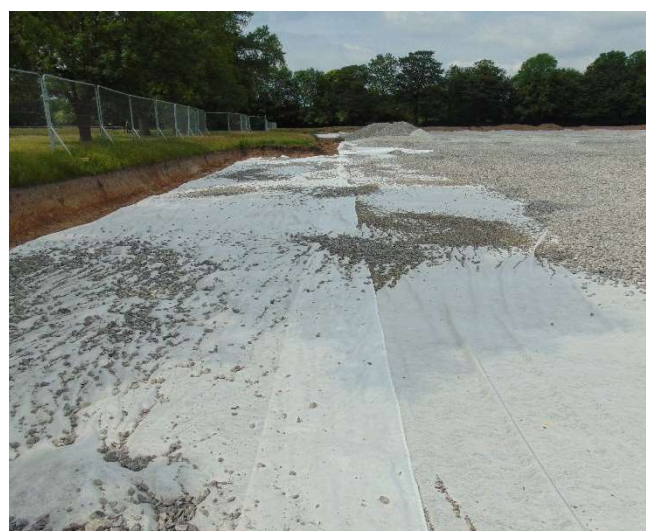
Fig. 6: Overlapping of Terrex sheet
