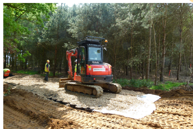
Can be trafficked immediately protecting the tree roots
