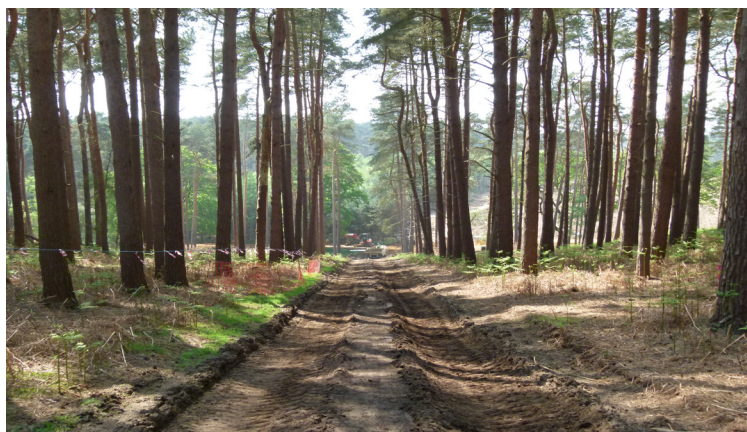
Rutting caused by traffic before the Abweb is placed
