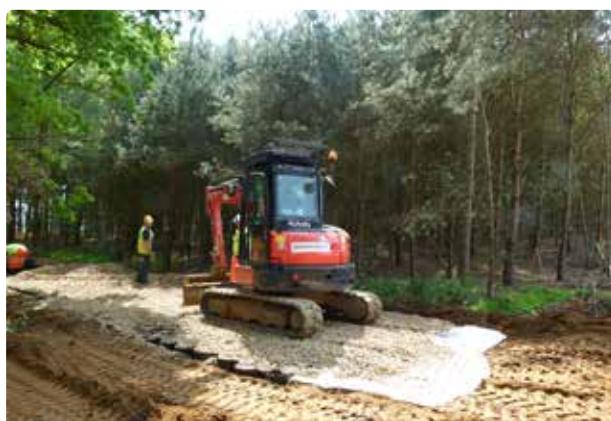
Infilling using filled area as a working platform
