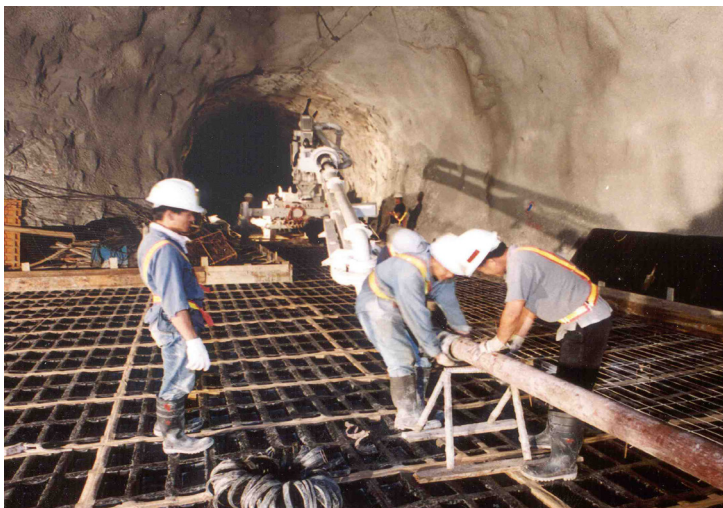
Preparing concrete pump to fill Cavidrain voids
