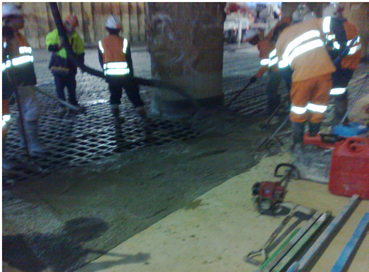
Straight-forward base slab construction
