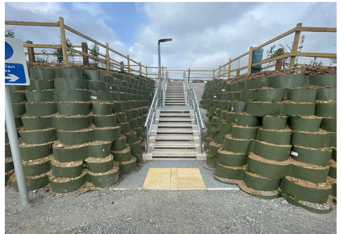
ABG Webwall forming 90° returns to accommodate a staircase
