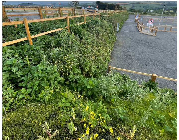
Vegetated Abslope EM section (foreground) adjoining with longer Webswall section
