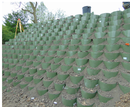
ABG gravity Webwall prior to planting and vegetation growth
