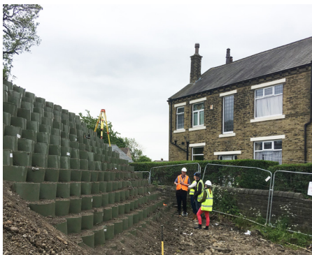
ABG gravity Webwall constructed around the constricted site boundary
