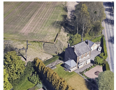
Aerial view of the built-in ABG gravity Webwall
