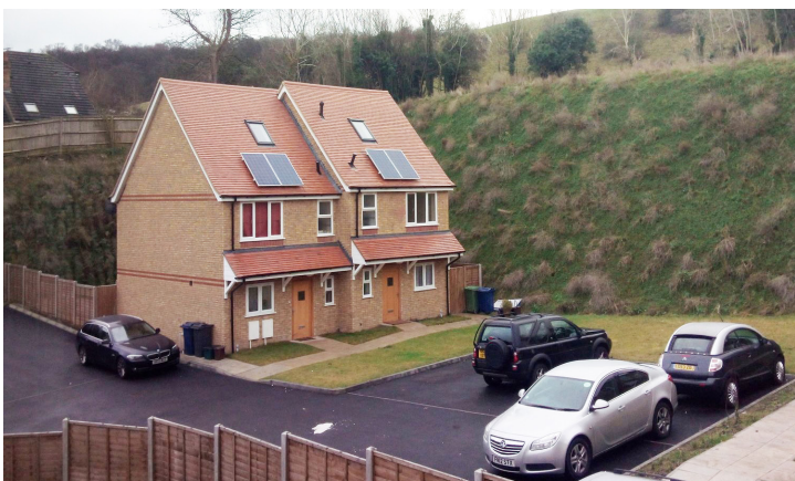
Webwall following initial grass coverage to provide a green finish
