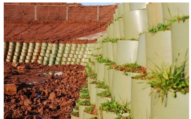
Fig. 14: Repeat process until design height is reached
