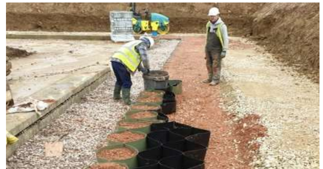
Fig. 5: Use of Chute to backfill front cells
