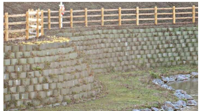
Fig. 15: Webwall external & internal curve spacings
