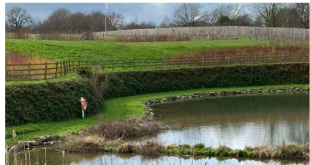
Fig. 16: Completed Webwall before and after planting. Planting required to provide protection against UV degradation.
