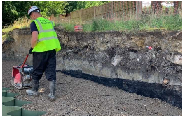
Fig. 8: Compact fill with roller or wacker plate
