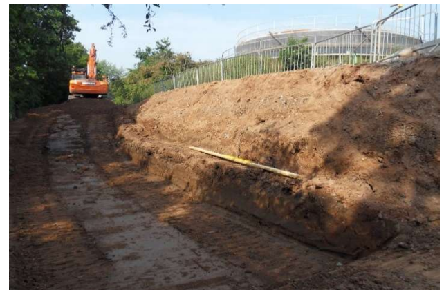
Fig. 2: Preparing site for Webwall installation
