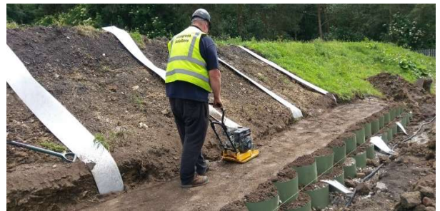
Fig. 12: Compact fill with roller or wacker plate
