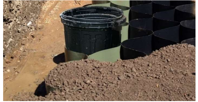
Fig. 7: Overfill base panels with granular fill
