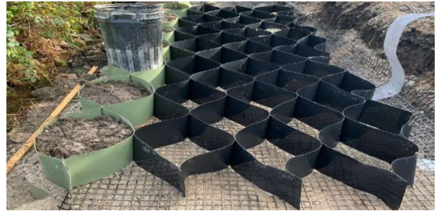
Fig. 11: First layer of Wall Construction ready for fill
