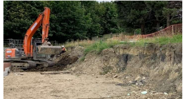
Fig. 4: Excavate a firm level footing
