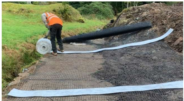
Fig. 10: Drainage and geogrid (where required)
